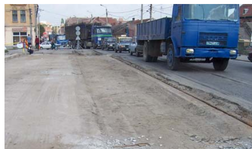
Photo 9 - Cleaned concrete plate
