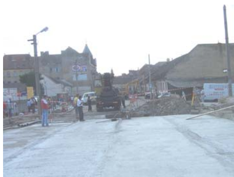
Photo 3 - Equalization concrete layer
