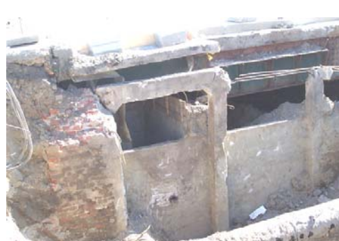
Photo 4 - Existing retaining wall
