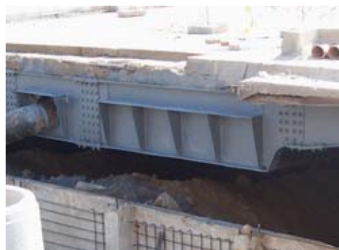
Photo 7 - Anticorrosive treatment on the girder and at the end of the bridge
