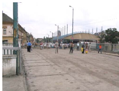
Photo 2 - Cleaned concrete plate
