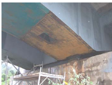
Photo 7 - Anticorrosive treatment on the girder and at the end of the bridge
