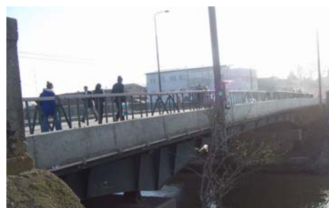
Photo 11 - New fence girder
