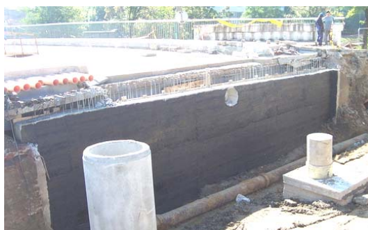
Photo 5 - New retaining wall
