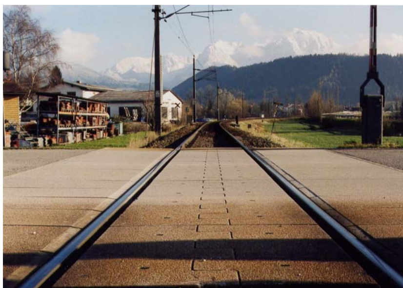
Figure 3: A highway-railway grade crossing with LeBODAN paving elements on the Linz-Selzthal railway line at Rossleiten
