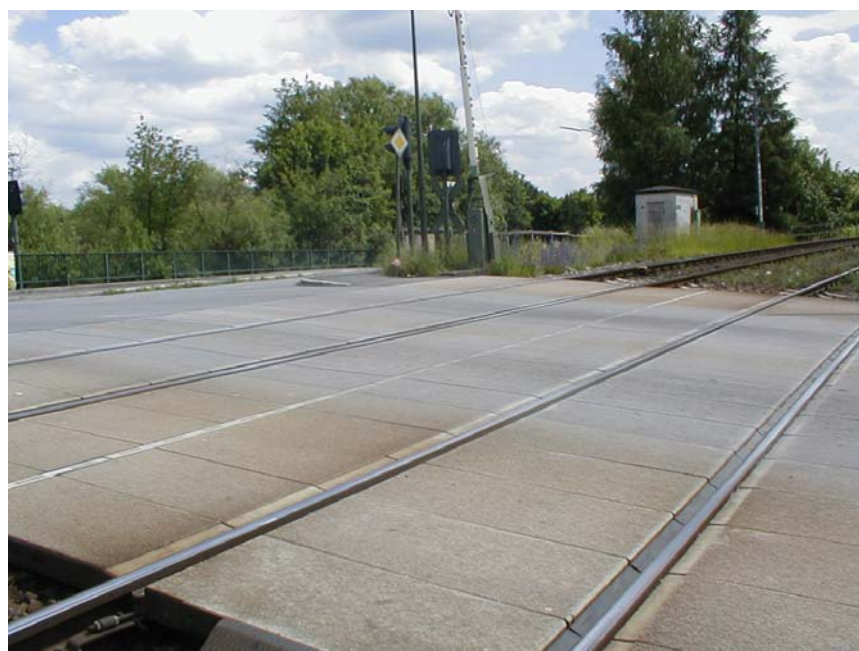
Figure 1: Polymer-bound paving elements in a double track railway line
