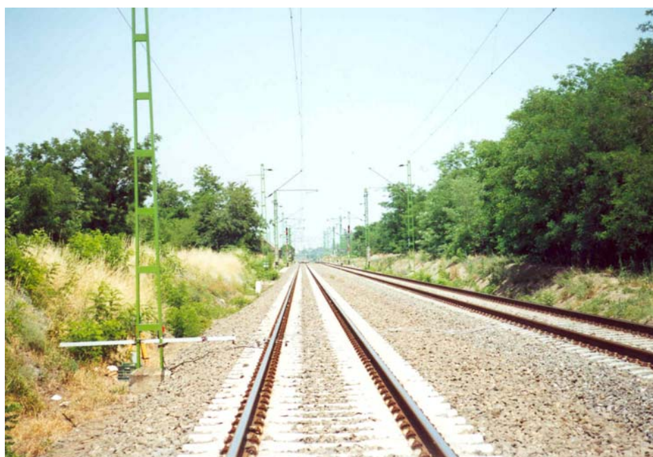
Figure 1: The site of the track measurements
