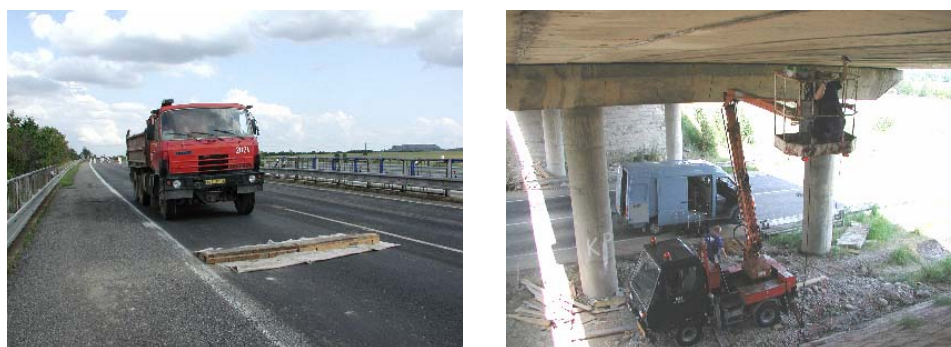
Fig. 4 – Testing on bridges
