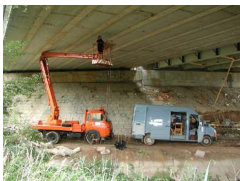
Fig. 6: Sensors placement process
