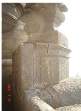
Figure 4. Detail of the detaching of pinnacles' structure from the battlement and view of the iron dowels on the back of the elements connecting the granite ashlars
