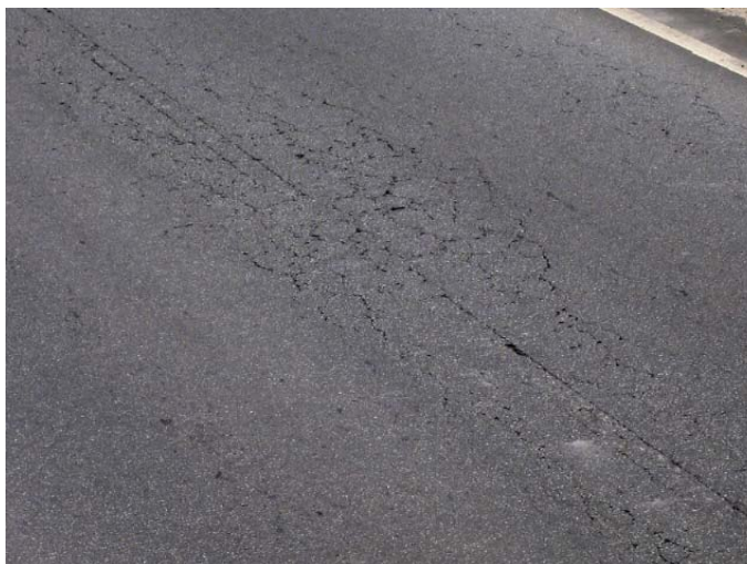
Photograph 1 – Cracked pavement (alligator cracking): pre-failure condition
