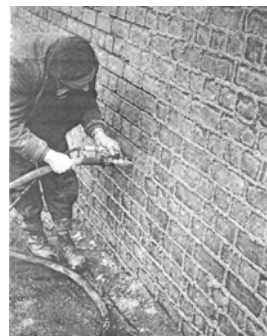
Figure 1. Repointing of the joints
