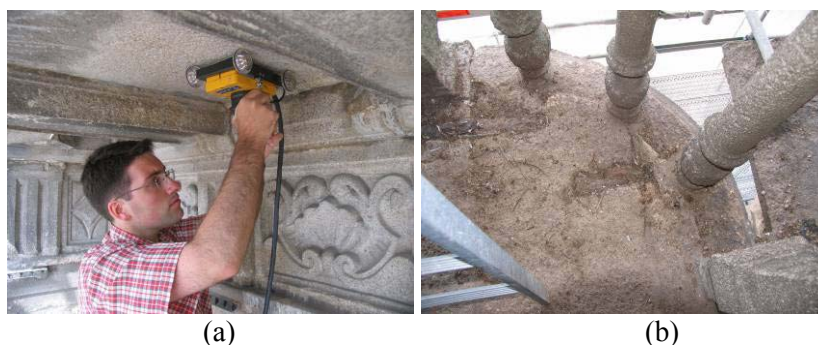
Figure 5. Central balcony: (a) inferior ribs of the slab, (b) steel connectors in the balcony's slab
