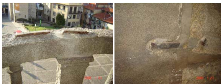
Figure 2. Details of the connection of the stones in the balcony's balustrade and between the ashlars of the slab
